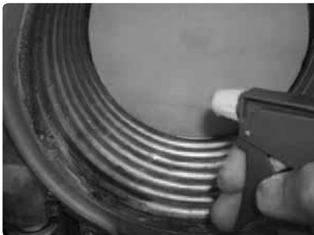
Figure 150 Cleaning the heat exchanger
