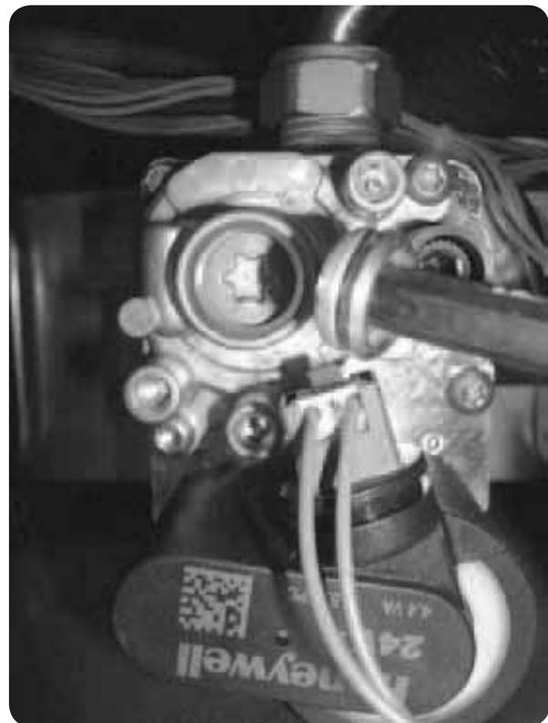
Figure 108 Remove T-40 cover cap with supplied Torx wrench for adjustment
