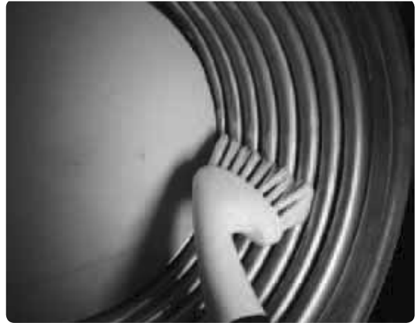
Figure 151 Cleaning the heat exchanger
