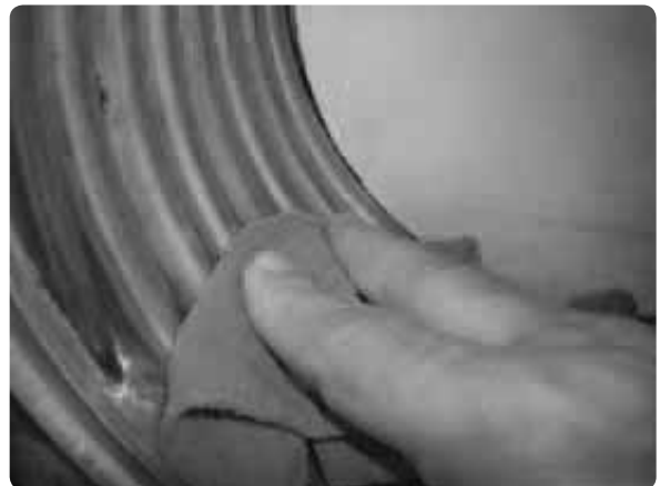
Figure 152 Cleaning the heat exchanger
