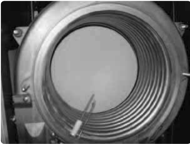
Figure 149 Inspecting and cleaning heat exchanger
