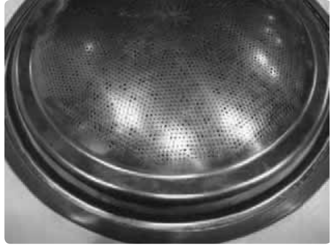
Figure 148 Inspecting exterior and cleaning the burner
