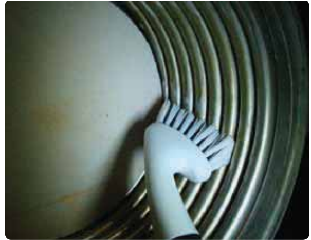
Figure 147 Cleaning the heat exchanger
