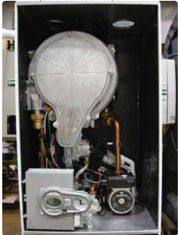
Figure 140 Boiler front panel removed (Combi 80/120 shown)
