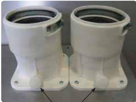
Figure 40 Vent (flue) and air adapters in place
