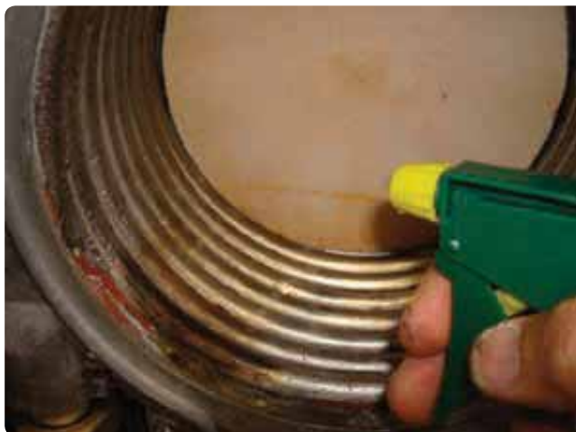
Figure 146 Cleaning the heat exchanger
