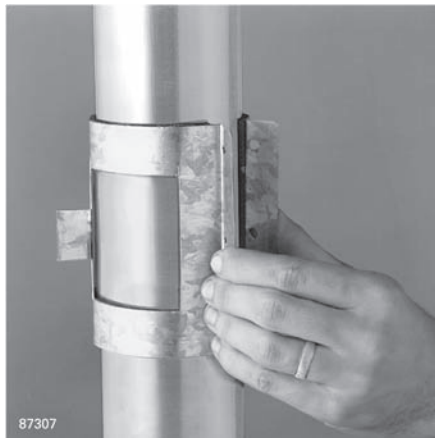
Figure 14 Install vent clamps on vent piping
